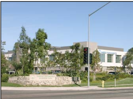
This office building demonstrates well-detailed elevations, ample landscaping and attractive monument signage.
