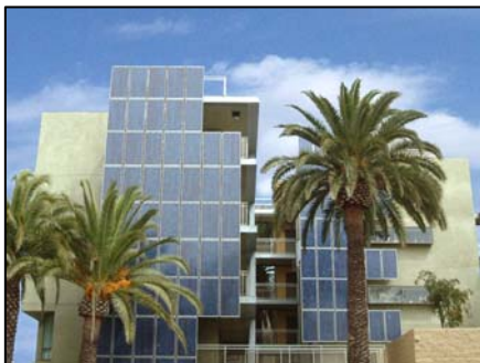
This active solar design can be complemented with passive techniques such as roof overhangs, window placement, and building orientation.
